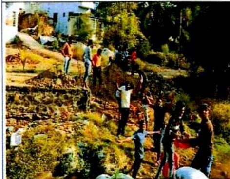
Construction of Vanrai Dam
