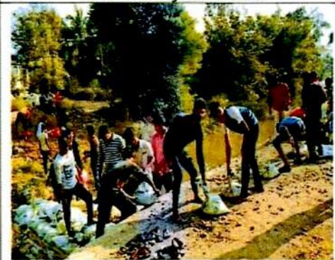
Construction of Vanrai Dam
