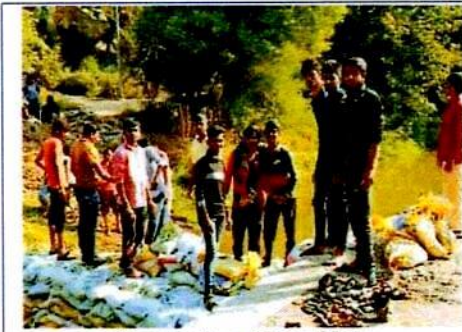
Construction of Vanrai Dam
